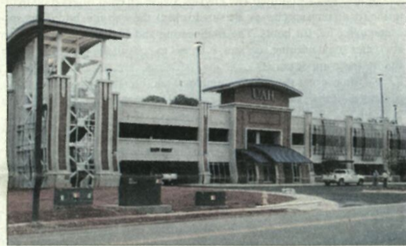
UAH's Intermodal Facility nears completion. (Photo by: Amber Rauschkolb)
