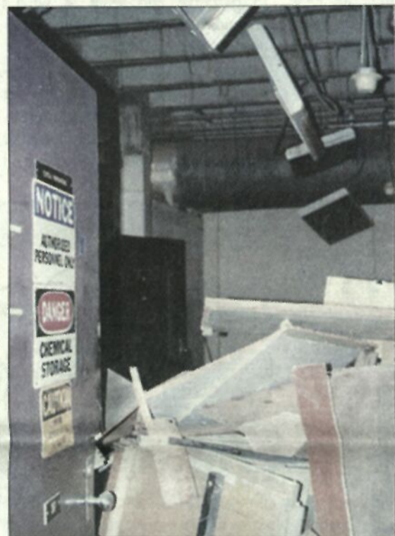
Gutting of Wilson Hall Continues (Photo by: Amber Rauschkolb)
