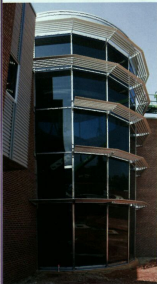
SWIRLL provides researchers with a new high-tech home for studying severe weather.
