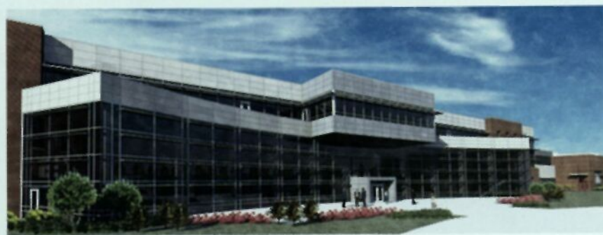
The new Student Services Building will open in the spring of 2016.
