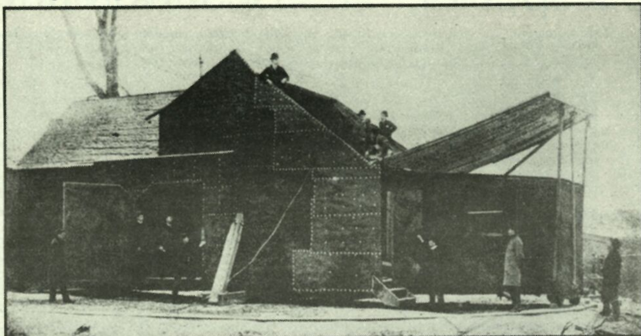
THE BLACK MARIA — Designed by Thomas Edison, the world's first film studio had a roof that swung open to allow for more light and sat on a circular track so that the entire studio could be turned to follow the sun. — Photo courtesy of NEA.
