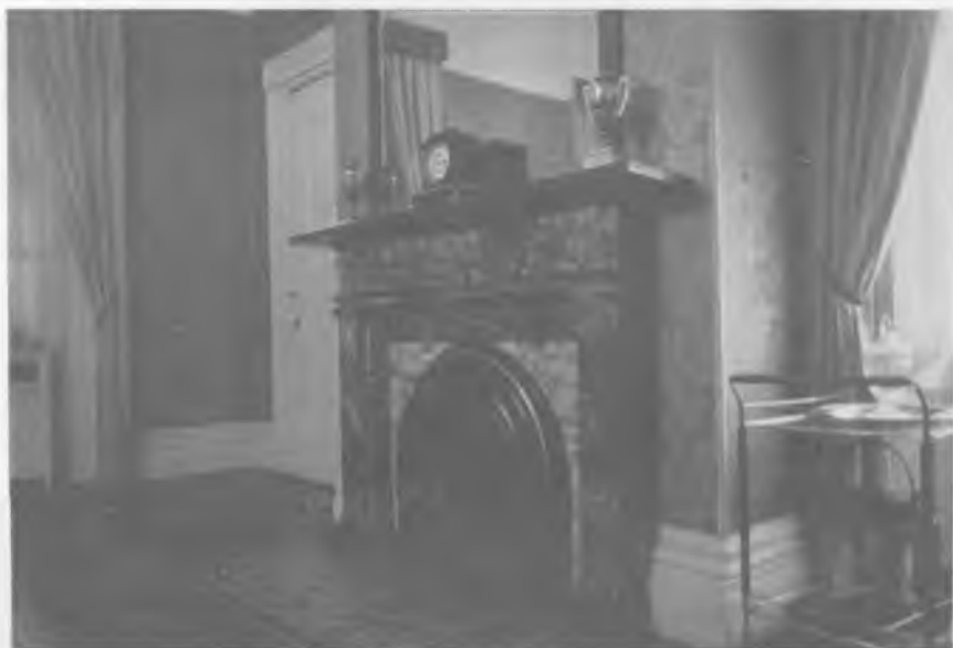
This black marble mantel in the dining room may have been in the house originally. Its design is Greek Revival and matches the corner pilasters of the house.
