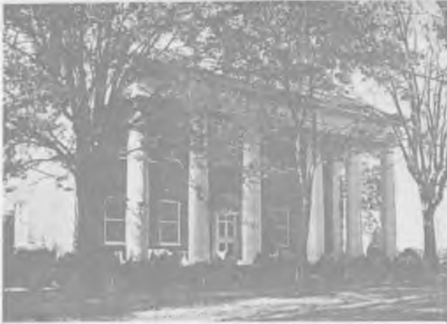
Belle Mina, with its six Doric columns, fanlight, and hipped roof, presents a different appearance from the Huntsville Bibb House. (Photograph from Ante-Bellum Mansions of Alabama by Ralph Hammond; photographs by the Author. Architectural Book Publishing Co., Inc. New York, 1951.)
