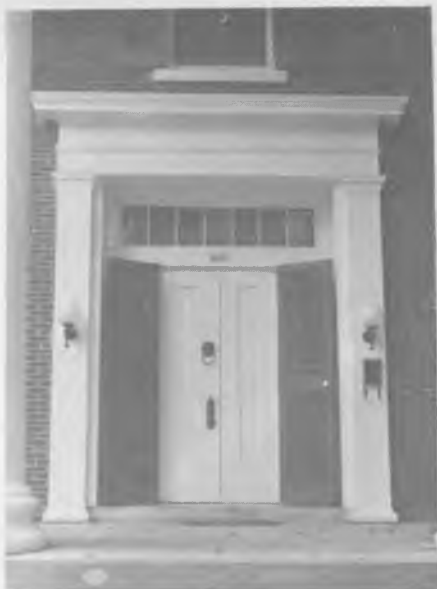
The oblong lights over the front door are Greek Revival, in contrast to the Federal fanlight over the front door of Bibb's Belmina house.
