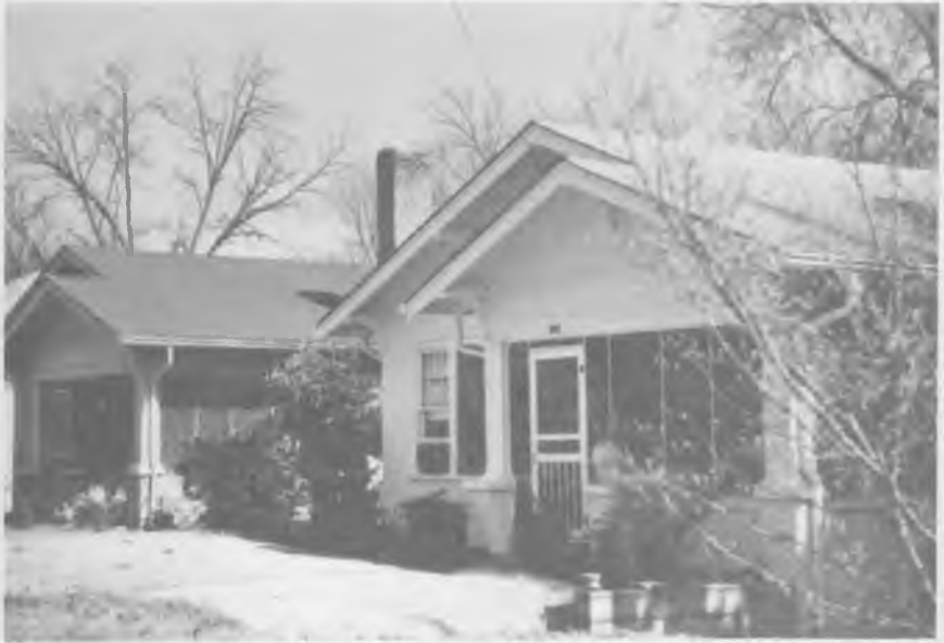
This pair of small identical bungalows at 430 and 432 Locust Avenue was built in 1923. They were probably built from stock plans on speculation, as many houses were in this boom period. The front porches were likely enclosed later, for screened front porches were not common in this period. The builder of these houses is unknown.
