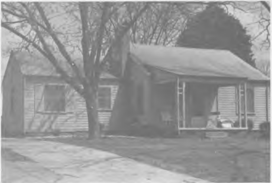
A large subdivision of houses similar to this one on Sewanee Road was built in the early 1940's during World War II to house Redstone and Huntsville Arsenal workers. Its style is derived from old New England cottages, except with a front porch added, and thus could be called a "Cape Cod Cottage" revival style.
