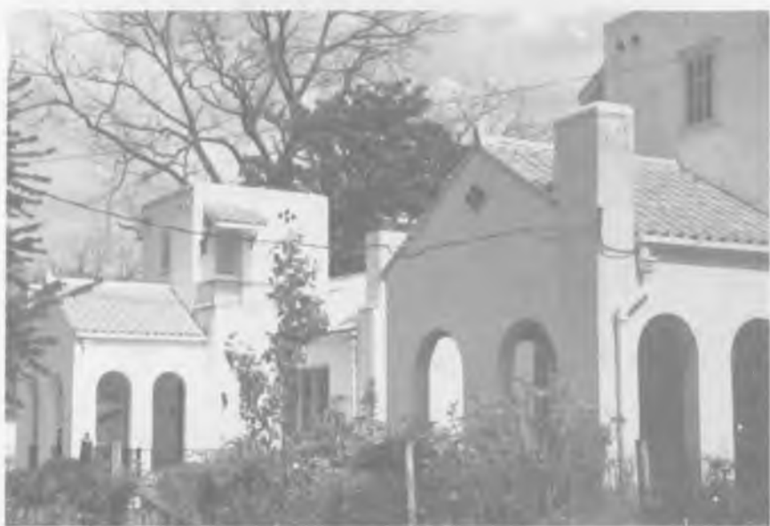
This pair of nearly-identical stuccoed houses at 136 and 138 Walker Avenue represent the Spanish Colonial Revival style, rare in Huntsville but very common in some other cities. They were built in 1929 by Harold Riggins. The ceramic pantile roofs are probably the 56-year-old originals. These small houses are unusually good examples of their style.
