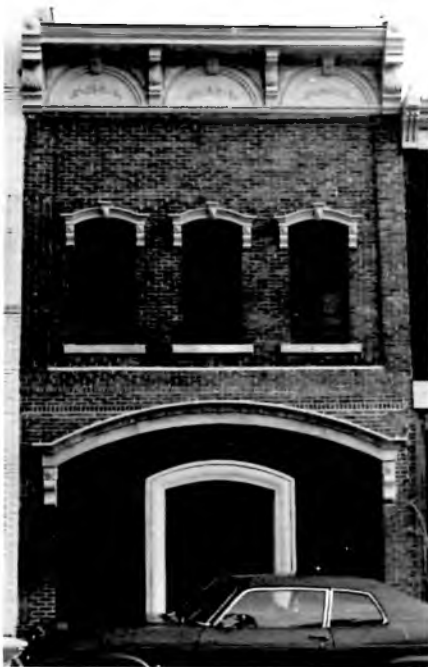
AFTER: A sensitive renovation has highlighted the surviving original elements, the cleaned brick and repainted cornice, while remodeling the ground floor to both harmonize with the existing design and provide a contemporary entrance.
