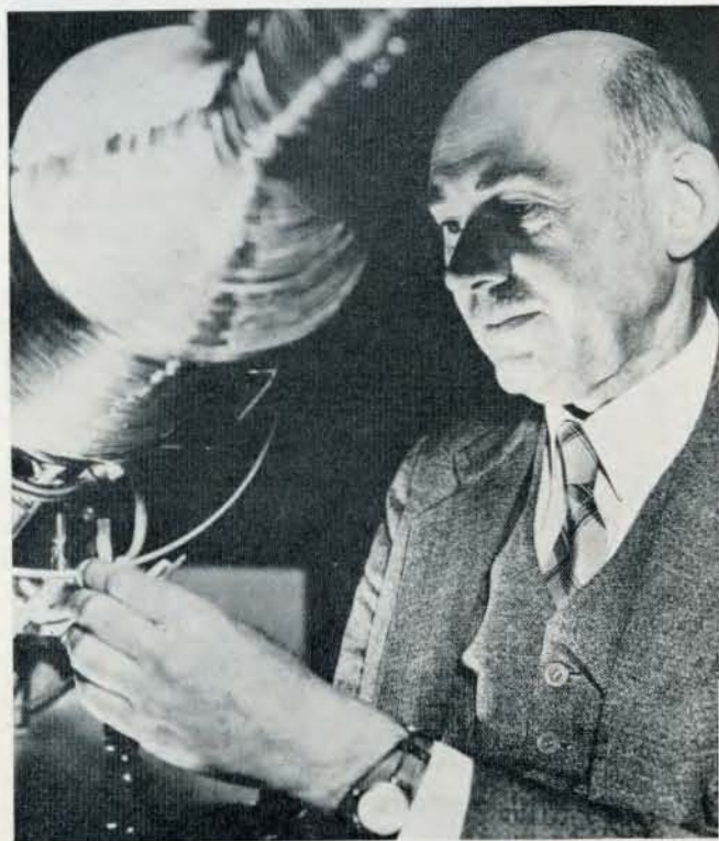
COPYRIGHT BY MRS. ROBERT H. GODDARD Dr. Robert H. Goddard making adjustments at the upper end of the rocket combustion chamber. Around the chamber are small coils of copper tubing for vaporizing liquid nitrogen in order to produce pressure for the fuel tanks and for operating controls. Pumps were used for the liquid fuels. Photographed in 1940.
