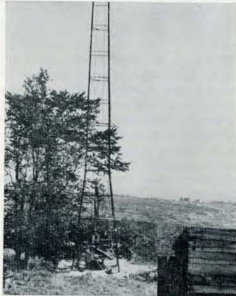
The launching tower and observation shelter at the Ward Farm, Auburn, Mass. Photograph taken on July 17, 1929.
