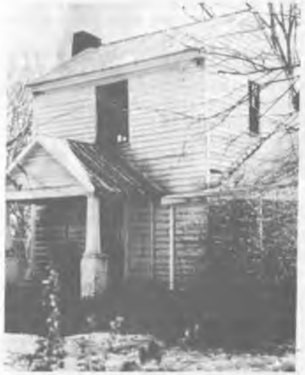
The Bannister Alley house
