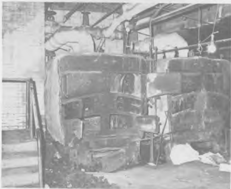
In the basement are found the coal-burning furnaces and the water pumps for sending water to the top floors.
