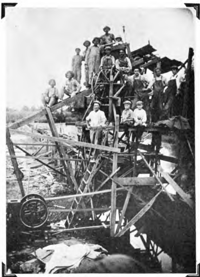
This old photograph shows the dam at New Market during construction. Fred Johnston is the man standing on the ladder in the center, immediately to his left is his son Ted, and Dorothea is the small figure at the top standing in the gravel car.
