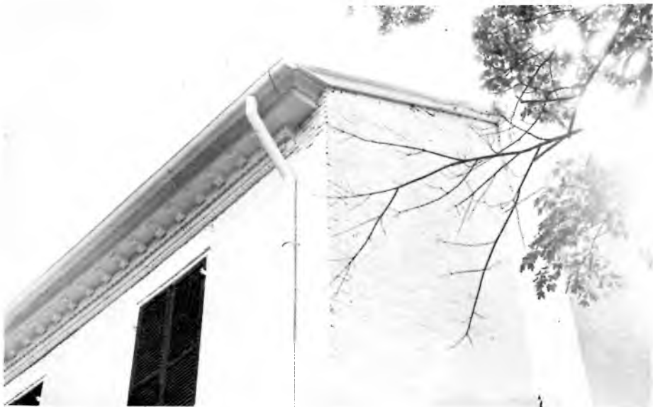
Cornice and gable wall of WEEDEN House.
