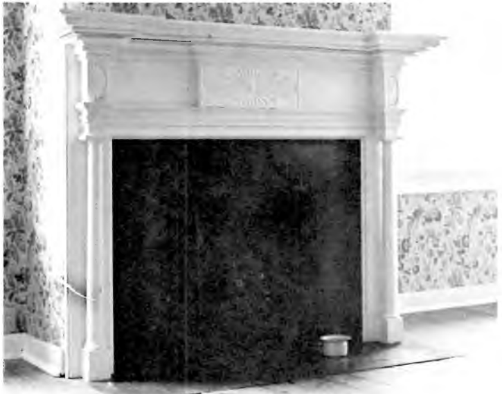
A Federal period mantel in the POPE House illustrating the use of Adamesque motifs such as sunburst designs, colonettes, and deep, flaring molds.
