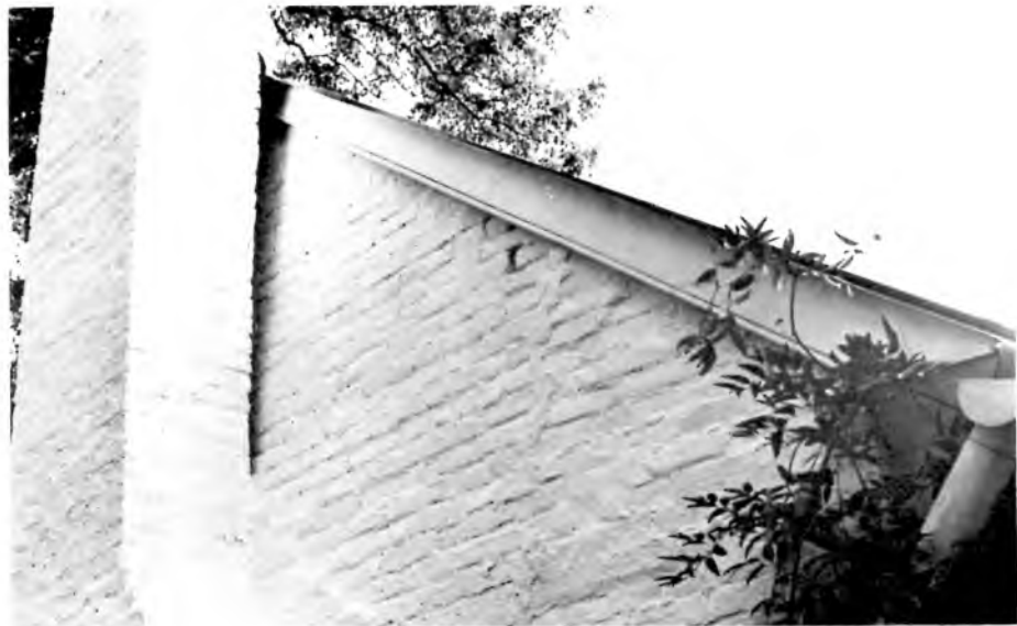
Rake-fascia on west service building of the POPE House.
