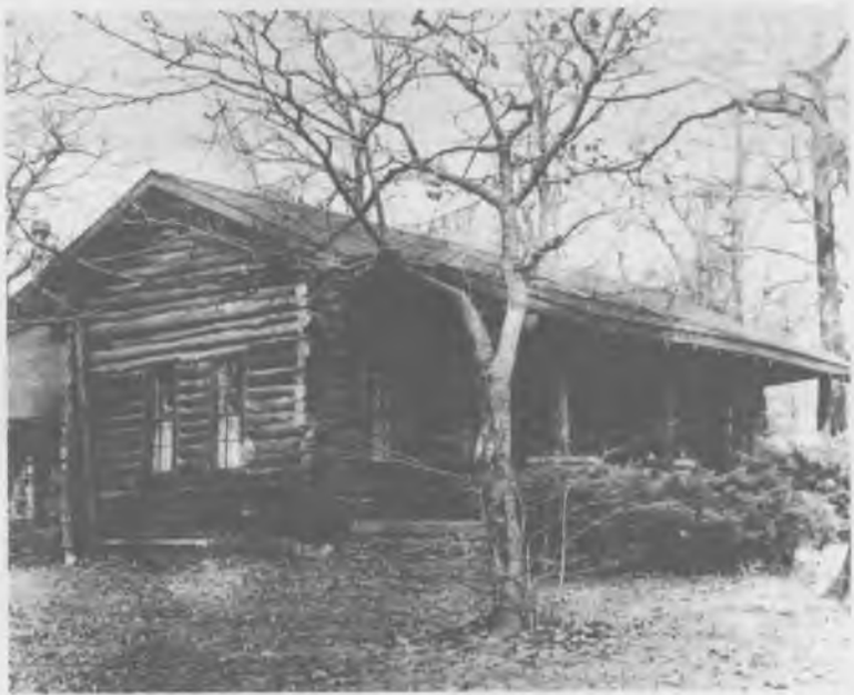
Old log house on Panorama Drive, Monte Sano, 1970 view.
