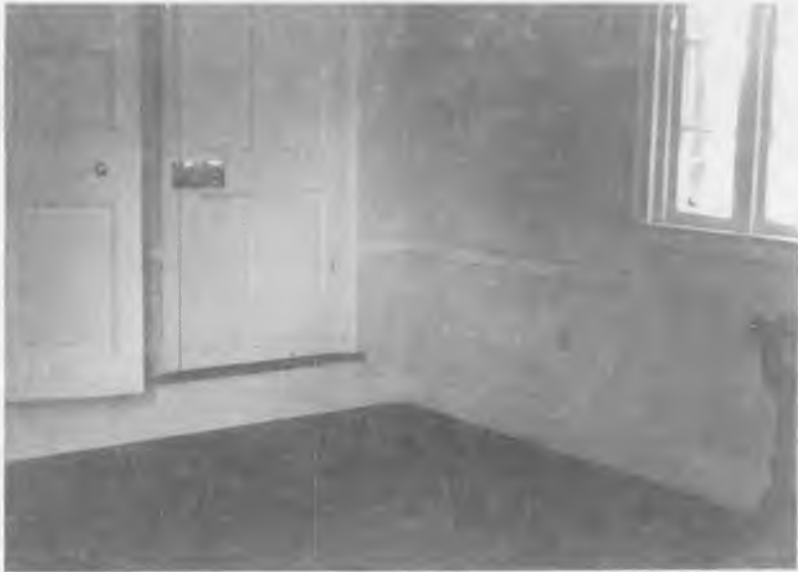
North bedroom after restoration. Note the raised closet door and hallway door (left), both opening to the higher-level floor of the Federal addition.
