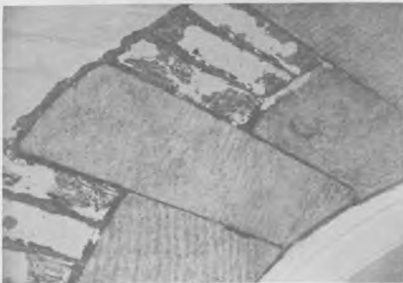
Detail of limestone and brick arch surrounding the Federal doorframe of the front entrance.
