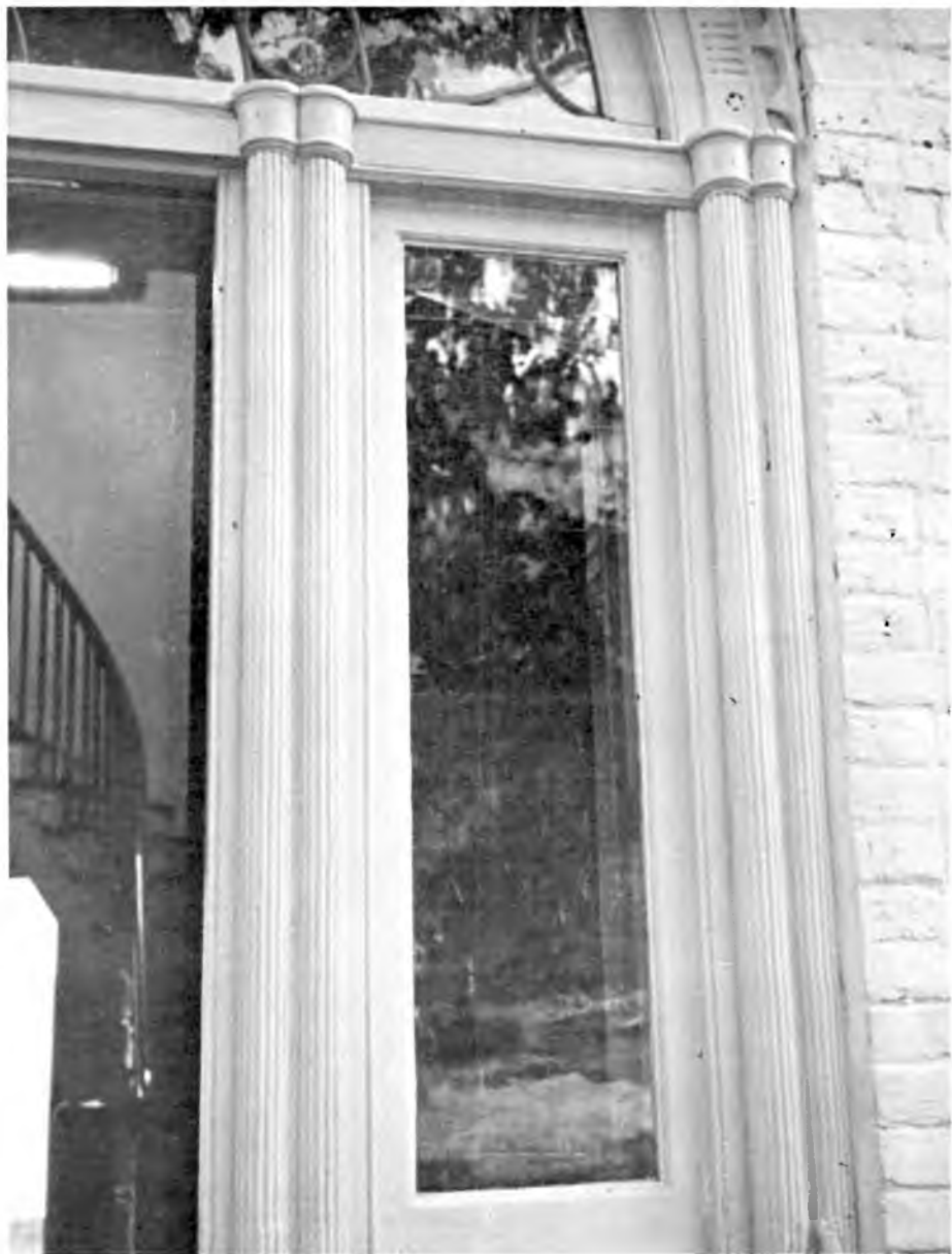
The sidelights of the front entry are flanked by extremely attenuated, reeded columns grouped in pairs. The leaded glass of the sidelights has been replaced.
