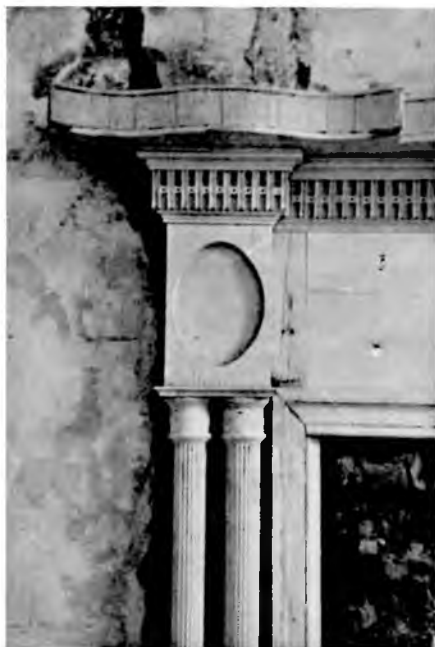
This mantel, located on the unrestored second floor of the Weeden House, displays the delicate reeding and fluting that were typical of Federal period decoration.
