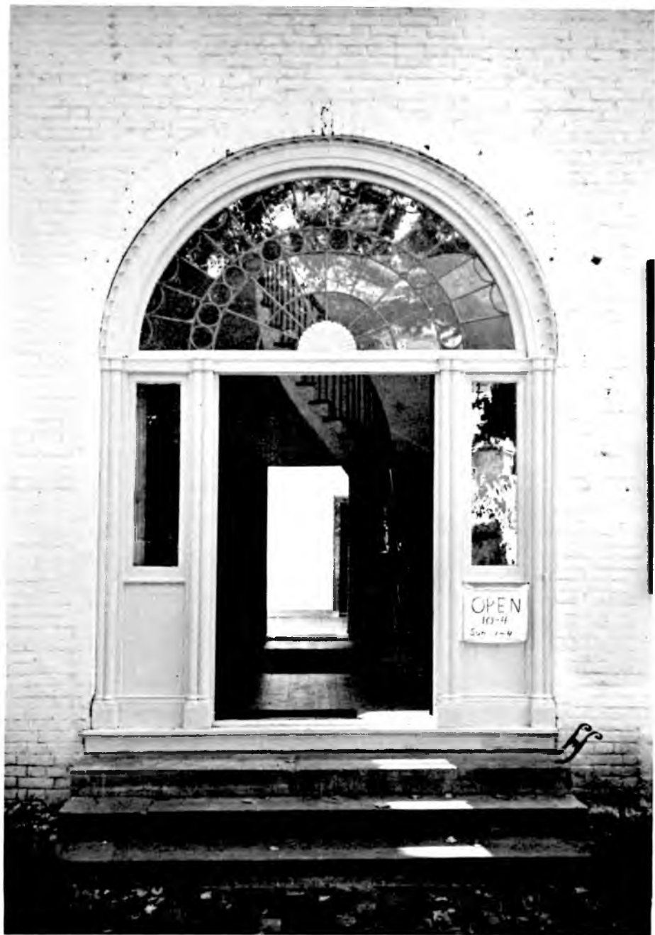
The front entry of the Weeden House
