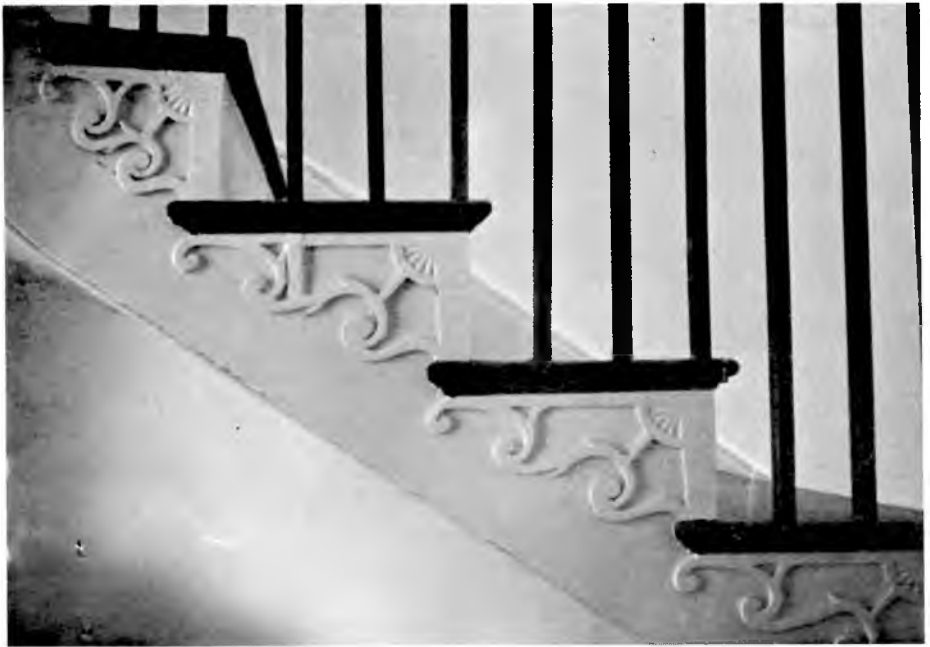
This detail of the stair scrolls shows how the pattern compresses as the stairway begins to curve.
