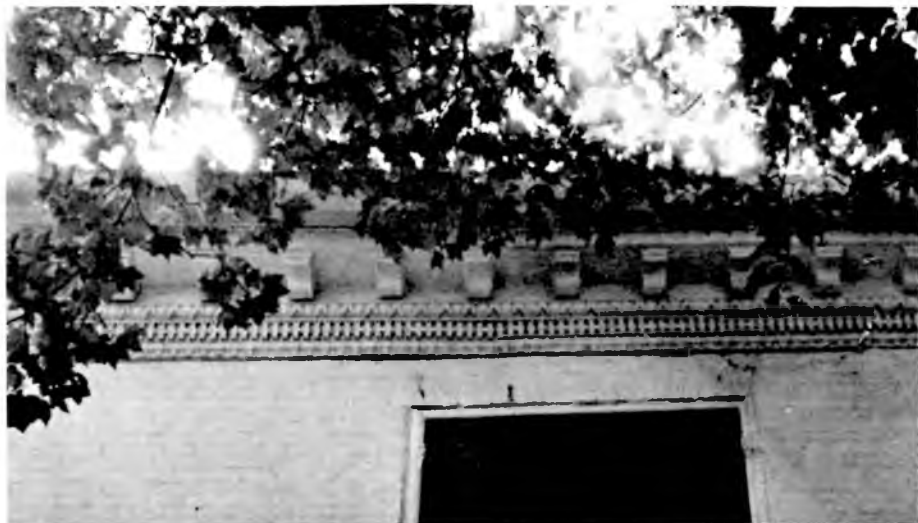
The roof cornice and frieze on the front facade.
