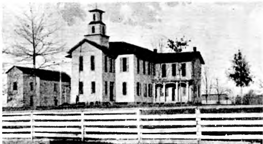
Huntsville's first public school building located on the site of the present East Clinton Street School.
