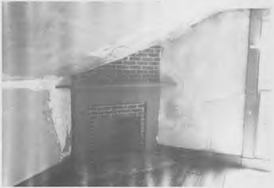
Corner fireplace in the unrestored east room upstairs. Note the sloping ceiling of the half-story level and the floor-to-ceiling length of the window.
