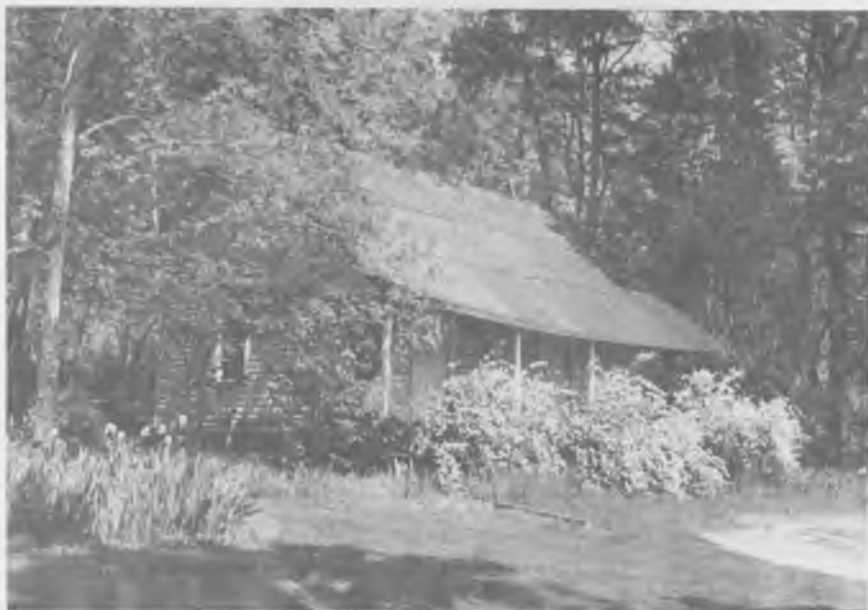
The two-room servants quarters cabin dates from the early days of the Christian plantation and possibly predates the house.
