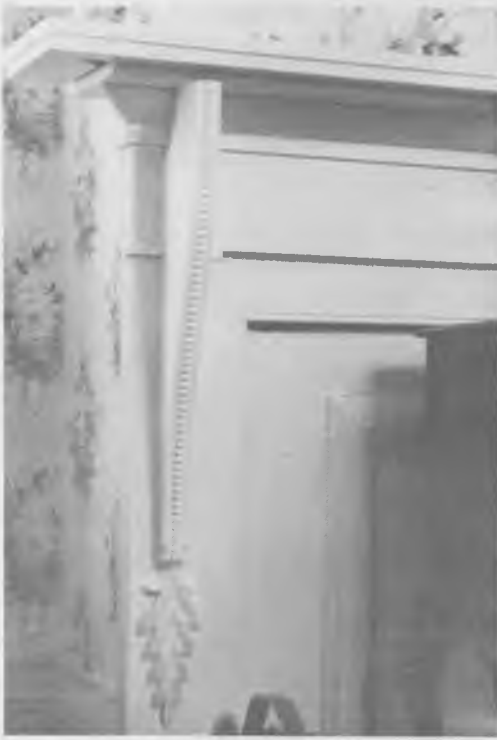
Detail of mantel in the dining room. Note the long bracket and carved leaf ornament added during the Victorian era to the plain Greek Revival style mantel.
