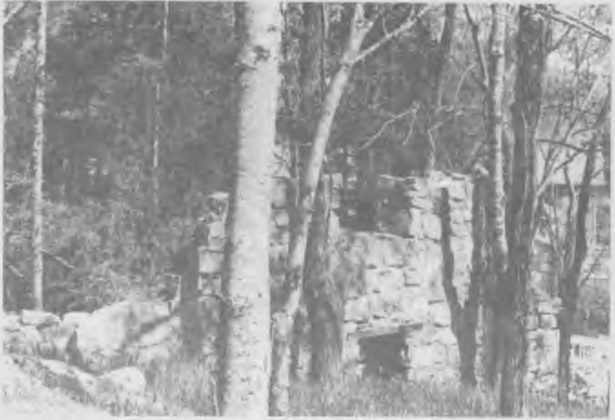
Part of the stone walls remain from the bottling house of Monte Sano Dairy.
