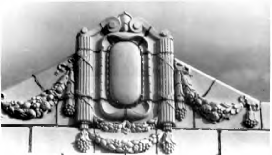
(19) (below) The Huntsville Times Building, 1928, Holmes Avenue. This Baroque-like cartouche contains classical elements such as floral swags and bundled reeds. It is made of the ancient ceramic material terra cotta ("cooked earth") that was revived and much-used in the latter 19th and early 20th century.
