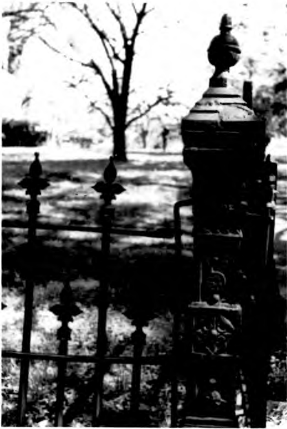
(9) Fence of cast and wrought iron elements combined, 310 Williams Avenue, date unknown, perhaps late 19th century. An example of decorative elements economically mass-produced by casting in a mould.
