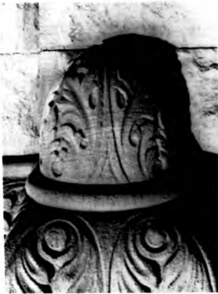
(10) Schiffman Building, 1895, East Side of Square. A fine, lively example of Romanesque Revival, where the idea seemed to be that absolutely nothing lines up or matches, with results that brighten the day of the observer. This is a bracket, carved in stone.
