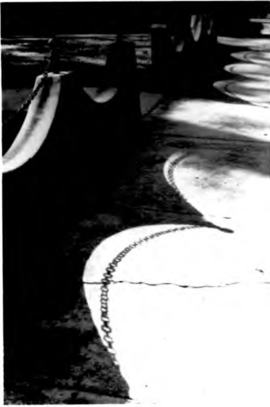
(18) Wall of concrete inverted arches and chain swags, McClung Avenue. Probably 19-teens, as is the house it fronts. A case of an attractive shadow cast by an architectural element.
