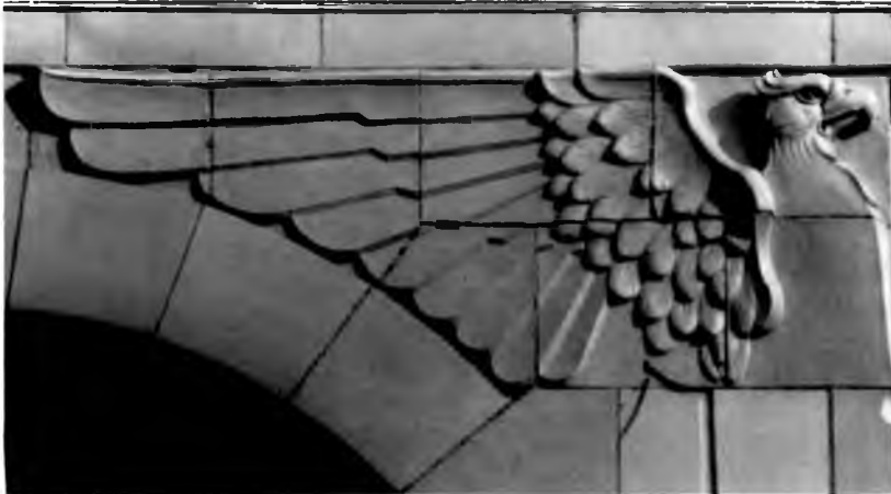
(21) The Huntsville Times Building, 1928. Four terra cotta eagles like this one guard the two entry arches. The Times Building was Huntsville’s first tall building, and used modified Gothic motifs in an Art Deco way to emphasize the building’s then-audacious twelve-story height.
