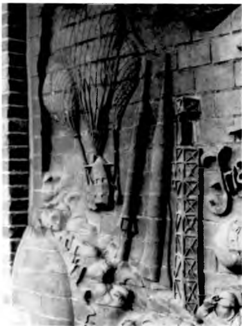
(25) General Shale Brick Co. Office, Whitesburg Drive, 1980's. A carved-brick mural produced by gouging the soft unbaked bricks into the desired profiles, firing them, and laying them up like a conventional brick wall (more tricky than it sounds).
