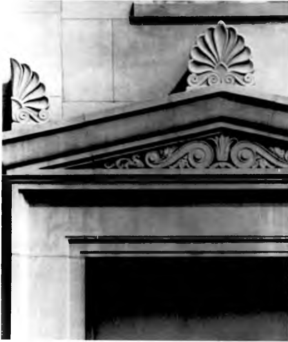
(22) Pediment, old 1932-35 post office (now Federal Court-house) on Holmes Avenue. The anthemion-like element at the corner and the peak of the Pediment is called an acroterion. The proportions and decoration of this Beaux-Arts Classical entry are derived from ancient Greek antecedents.
