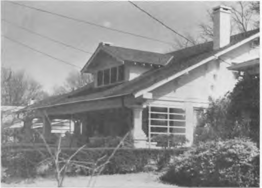
9. This 418 Locust Avenue 1922 bungalow exhibits the Swiss influence (long, low swooping roof, large dormer, stucco, false half-timber) but not in a literal manner.(3) Notice the "missing" porch columns - a deliberate design feature. It would be an error to "replace" them. This house was built by Fisk & Hopper, contractors. Its design probably came from a "bungalow book" of stock plans.
