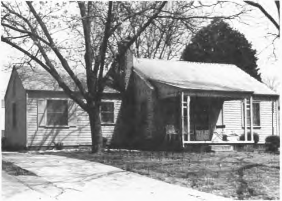
13. A large subdivision of houses similar to this one on Sewanee Road were built in the early 1940's during World War II to house Redstone and Huntsville Arsenal workers. Its style is derived from old New England cottages, except with a front porch added, and thus could be called a "Cape Cod Cottage" revival style.
