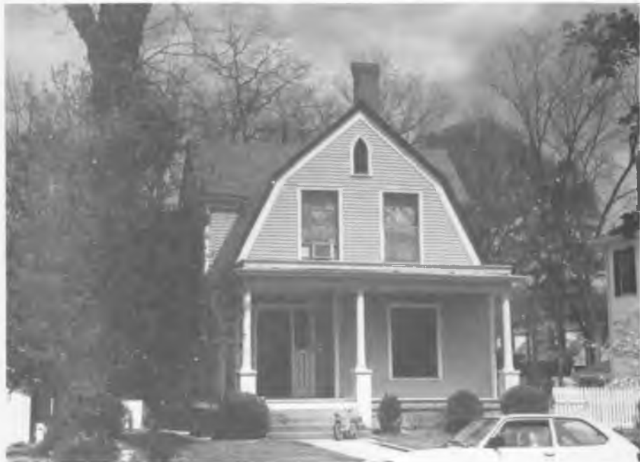
2. This 1901 house at 603 Franklin Street by the architect Herbert Cowell has a Dutch-Colonial Revival gambrel roof combined with late-Victorian massing (vertical, narrow, irregular). A small "Gothic" vent is in the gable. The windows are quite wide and squarish in proportion, unlike those in the Victorian styles. A balustrade once ran along its porch roof, as evidenced by the base for it, and there may have been a balustrade also at the porch floor level that ran between the masonry piers which support the porch columns.
