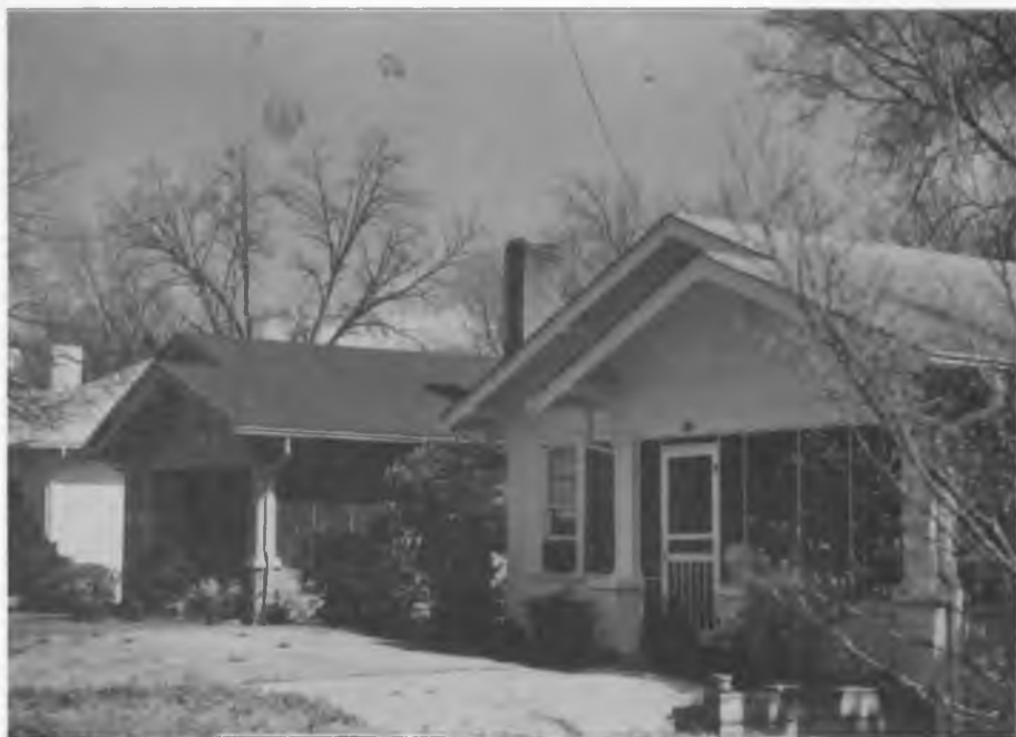
This pair of small identical bungalows at 430 & 432 Locust Ave. were built in 1923. They were probably built from stock plans on speculation, as many houses were in this boom period. The front porches were likely enclosed later, for screened front porches were not common in this period. The builder of these houses is unknown.
