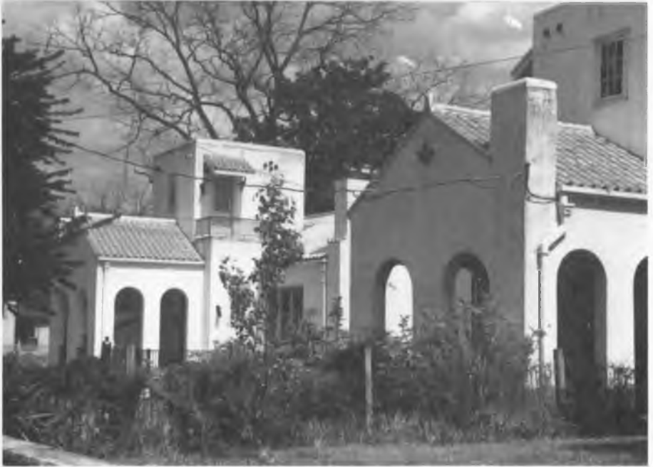
11. This pair of nearly-identical stuccoed houses at 136 & 138 Walker Avenue represent the Spanish Colonial Revival style, rare in Huntsville but very common in some other cities. They were built in 1929 by Harold Riggins. The ceramic pan-tile roofs are probably the 56 year-old originals. These small houses are unusually good examples of their style.
