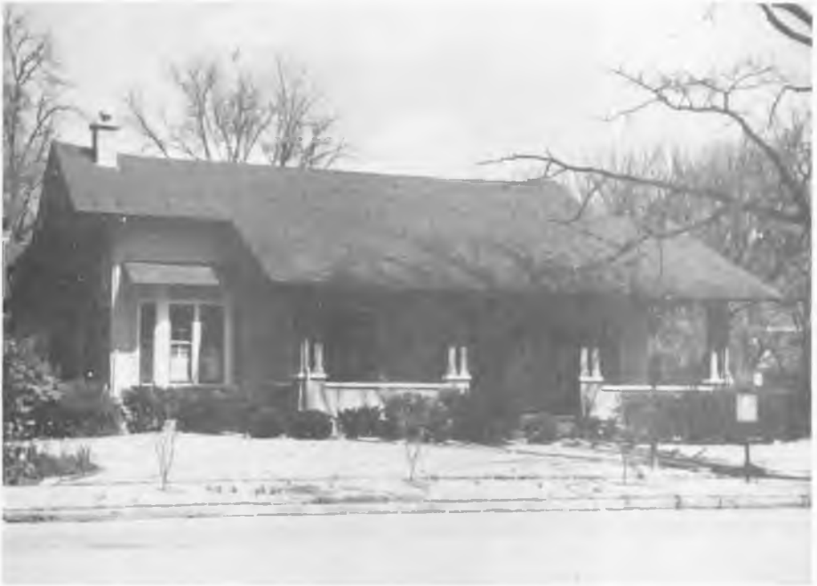
5. This fine early bungalow at 531 Franklin Street was designed in 1909 by the Huntsville architect Edgar Love. Notice the "kick" of the roof-ridge ends - a refinement found in at least one other Huntsville bungalow. The zig-zag roof and bay window give this bungalow an informal and welcoming air.
