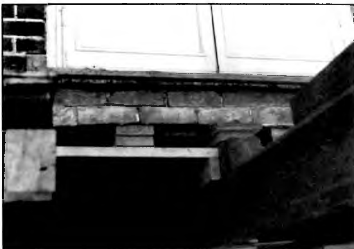
Detail of steel pins and wooden intermediate blocking to support the solid brick walls at close intervals. No cracking occurred due to the move.
