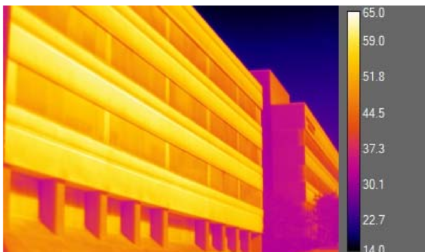
Image 1. IR image comparing the east facing side of Cramer Hall with a South facing wall.
