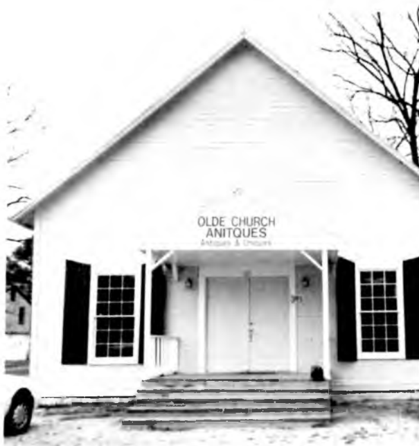
Mill Village church ca. 1907 on Humes Avenue lives on as an antique store. Store owners stripped and preserved original exterior and interior. Roof was repainted. Shutters are new but reproduce originals.
