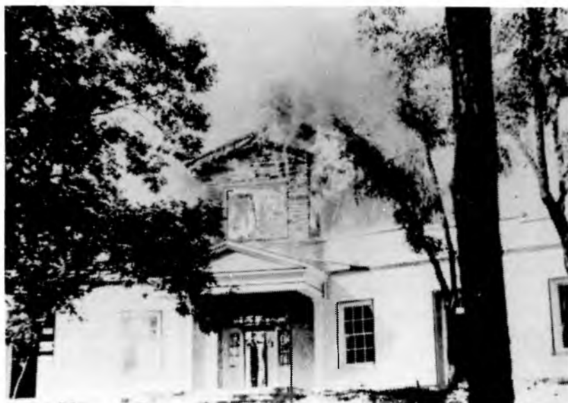
Dr. Burritt's first house on fire, June 6, 1946.
