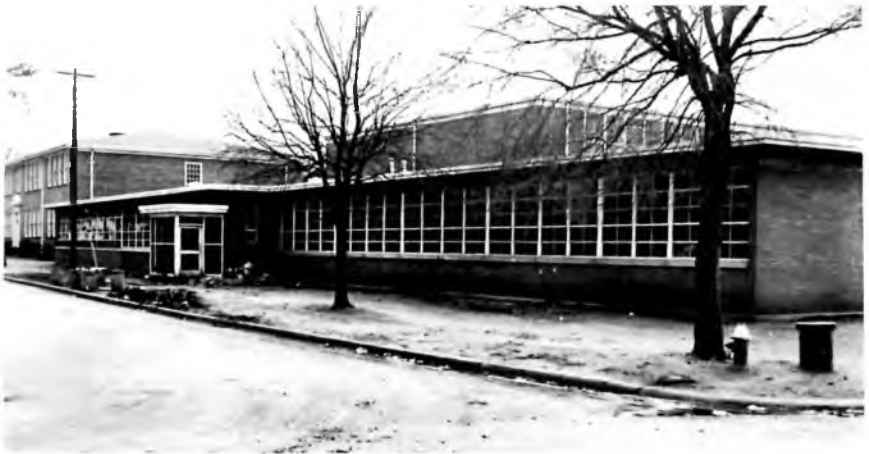
William H. Council High School building in 1994 used by Arts Council groups
