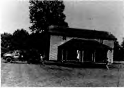
The Balch House relocation in 1985. This was the first structure moved to the Historic Park
