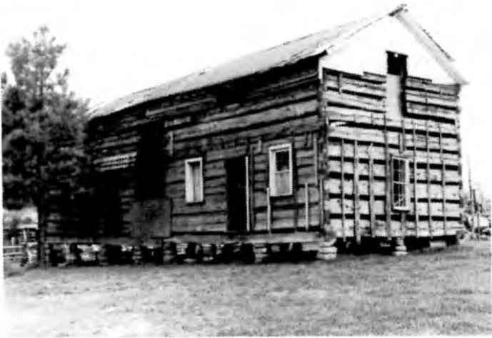
Above: James A. Meals house on site at Burritt Museum. The clapboard siding has been removed to determine which logs need to be replaced. 1994.
