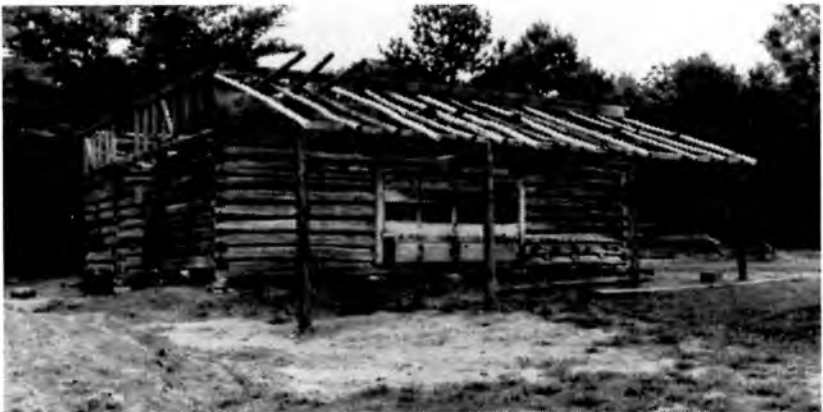
Barn in progress, 1993.
