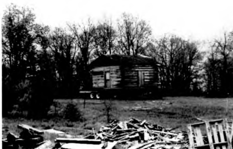
Above: The Smith-Williams House being moved from the parking lot area to its present location in the Historic Park. August, 1991.
