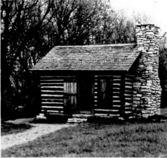
The Gardiner Cabin soon after restoration. Note the stacked rock limestone chimney. April, 1991
