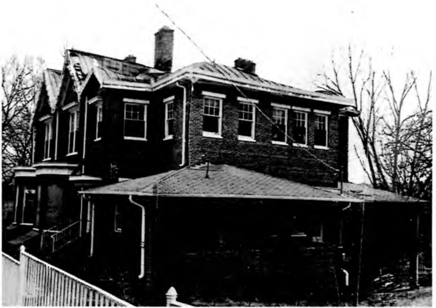
BEFORE Picture taken in 1974. Includes a 1960s carport and kitchen addition. (Taken after the 1973 fire.)
