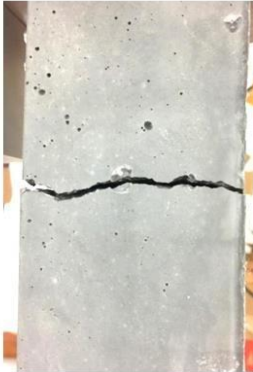
Figure 2.1 Plain Concrete Fracture in Tension [40].
