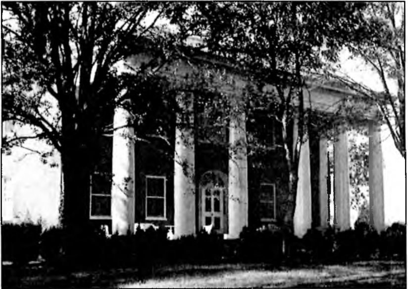
Front view showing Portico. From "Ante-bellum Mansions of Alabama."
