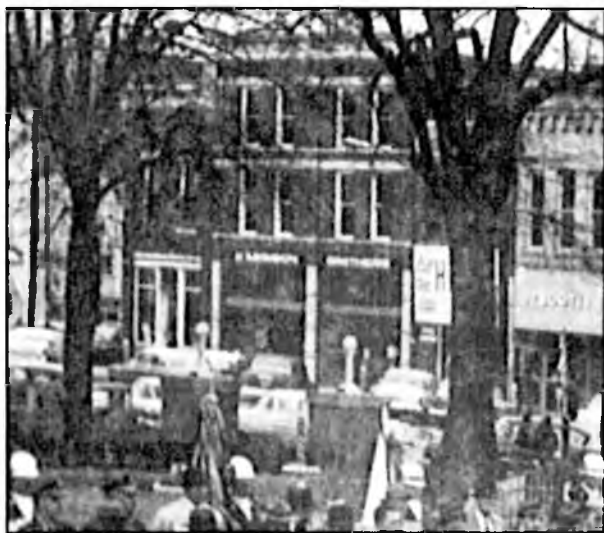
Hundley Building on corner. Ca. 1960 parade, looking SE.
