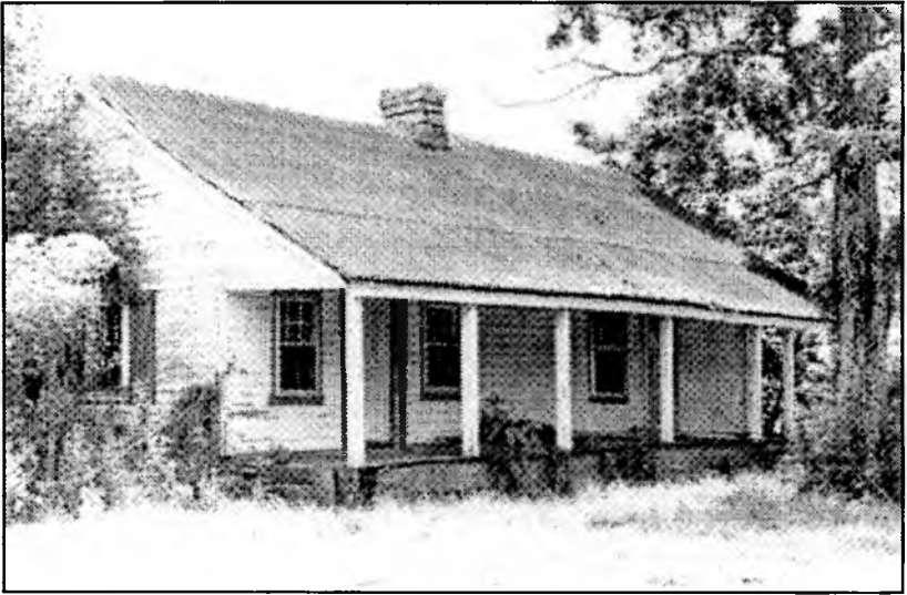
Fig. 3 First generation saddlebag house, modernized, Poplar Ridge Road, south of Cherry Tree Road, Madison County. Courtesy Debra Miller.
