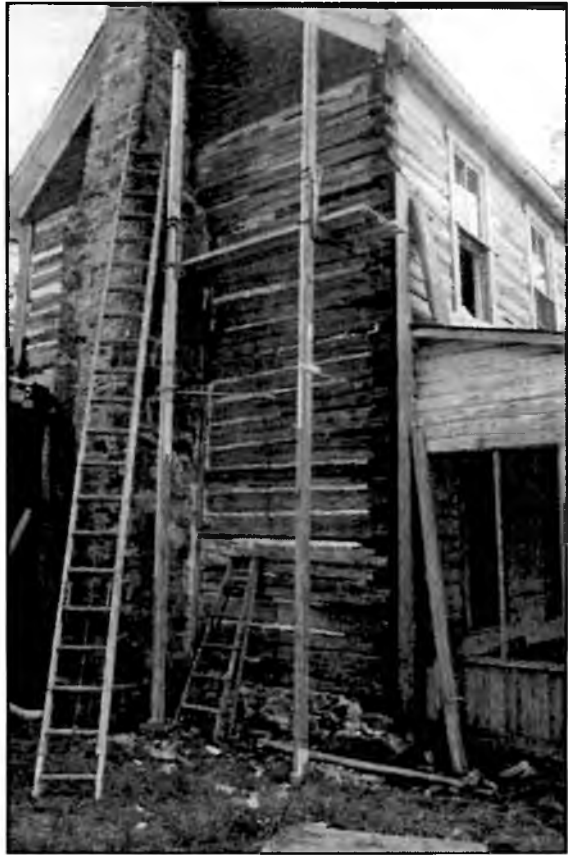
Fig. 7 Exterior of Cabaniss-Ezell House, late 1980s.
