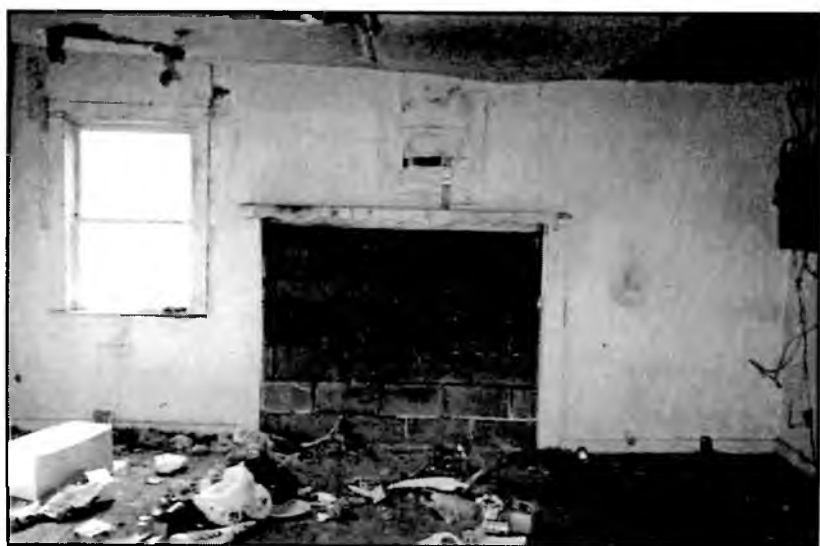
Fig. 3 Hollingsworth-Allen House fireplace, November 1994 & December 1995.
