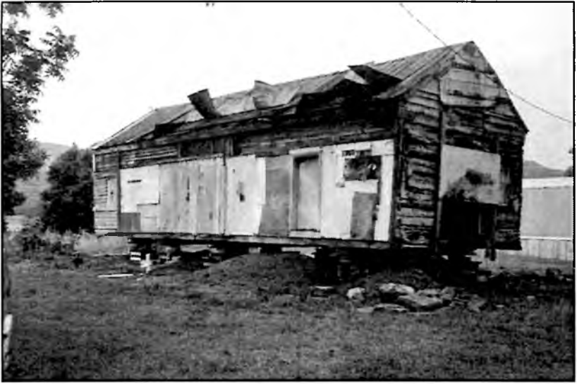
Fig. 5 Hollingsworth-Allen House in process of being raised, May 1995.
