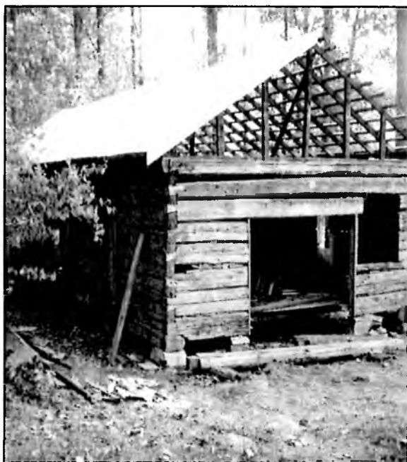
Fig. 7 Replacing the tin roof, Hollingsworth-Allen House, September 1995. Courtesy Jan Allen.
