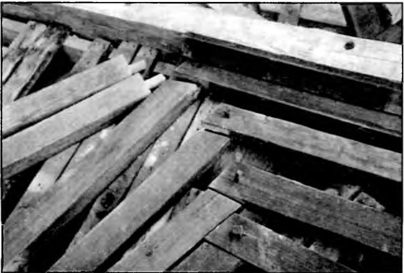
Fig. 4 Roof rafters, disassembled, Hollingsworth-Allen House, June 1995.
