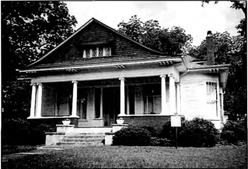
Fig.2 Front view of Johnson-Burwell Bungalow. Courtesy Jackson P. Burwell, P.C.
