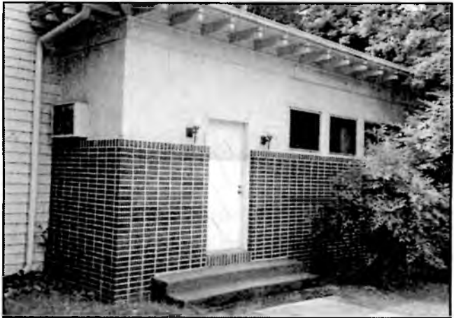
Fig.2 Front porch before restoration. Courtesy David Bowman.
