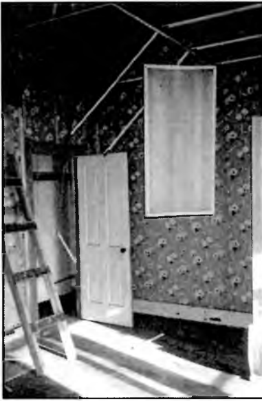
Fig.7 Removal process of light fixture and electrical conduits. Courtesy David Bowman.
