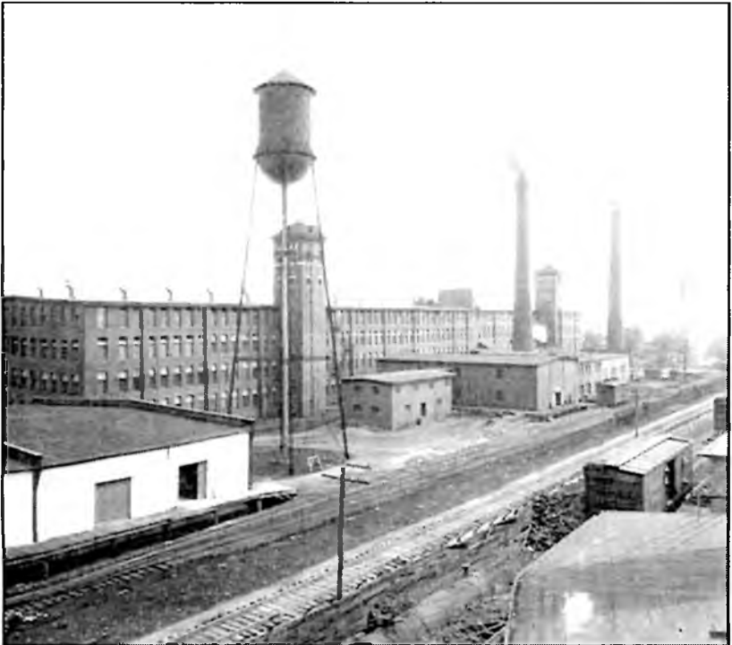
Dallas Mill Water Tower. Courtesy Huntsville Public Library.
