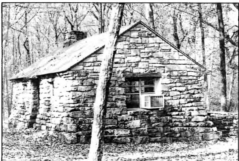
Fig.8 Cabin at Monte Sano State Park before renovation. Notice windows. Courtesy Kent Wilborn.
