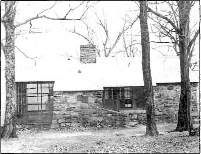
Fig.6 Before renovation: notice trim and light roof. Courtesy Kent Wilborn.
