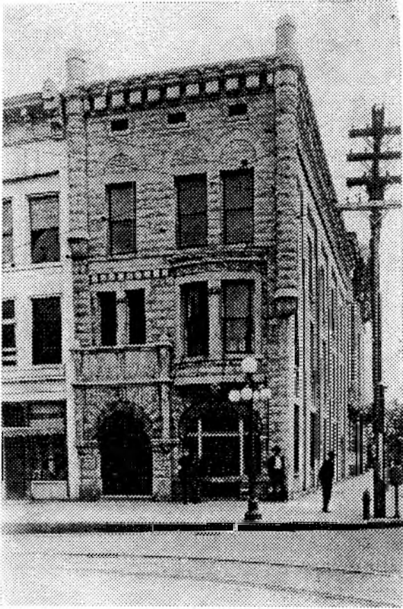
Fig.1 The Schiffman Building, corner of East Side Square and Eustis Street. Notice the trolley tracks in this undated photograph. Courtesy Huntsville/Madison County Public Library.
