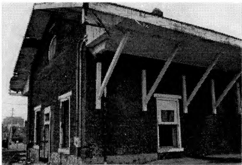
Fig.3 Office end of freight depot, October 1998. Notice Courthouse in background.
