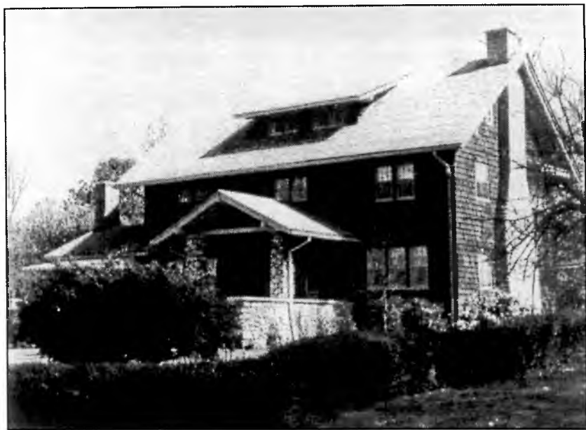
Fig.6 The 1914 house at 612 East Holmes Avenue could be termed a Swiss-style bungalow. It bears a strong family resemblance to many 17th and 18th century Swiss rural houses, with its use of fieldstone, natural wood shingles, and steep gabled roof. The wide, low shed-roofed dormer is also found on old Swiss houses (Smith 52,53). These Swiss forms, including the use of rough-cast stucco and false half-timber, are found on many bungalows, and it would be fair to say that old Swiss houses were a major influence on the bungalow style. Courtesy Lynn Jones.
