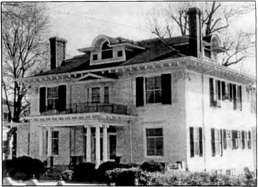
Fig. 4 A free adaptation of the Colonial Revival style is represented in this 1907 house at 418 McClung Avenue. While the basic design is technically Colonial Revival (boxy shape, hipped roof, fanlighted and sidelighted entry, modillions, Palladian dormer, sash-blinds, etc.), the proportions are vastly different from the late-Georgian ancestors of this fine house. The roof eaves are about three feet wide—over three times as wide as those of an 18th century Georgian house. The modillions at the eaves are gargantuan in comparison to 18th century ones. On the other hand, the clapboards are extremely narrow, about one-third as wide as in the Georgian period. All this disregard for academic correctness comes off splendidly, and the result is an excellent early 20th century house instead of a pale copy of an 18th century one. Courtesy Lynn Jones.
