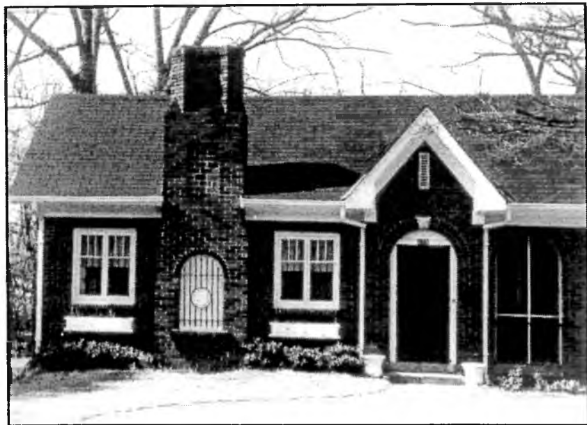
Fig. 12 The sculptural chimney, dark brick, and steep roof denote this house as being of the English Cottage style. This house at 609 Randolph Avenue was built circa 1930. This style is frequently referred to as Tudor. The Old House Journal feels that this term should be restricted to half-timber versions of this English Renaissance Revival style. Courtesy Lynn Jones.
