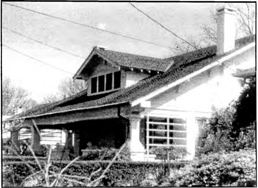
Fig. 9 The Swiss influence was strong in many bungalows. The 1922 bungalow at 418 Locust Avenue exhibits the Swiss influence (long, low swooping roof, large dormer, stucco, false half-timber), but not in a literal manner (Smith 52,53). Notice the missing porch columns—a deliberate design feature. It would be an error to replace them. This house was built by Fisk & Hopper, contractors. Its design probably came from a bungalow book of stock plans. Courtesy Lynn Jones.
