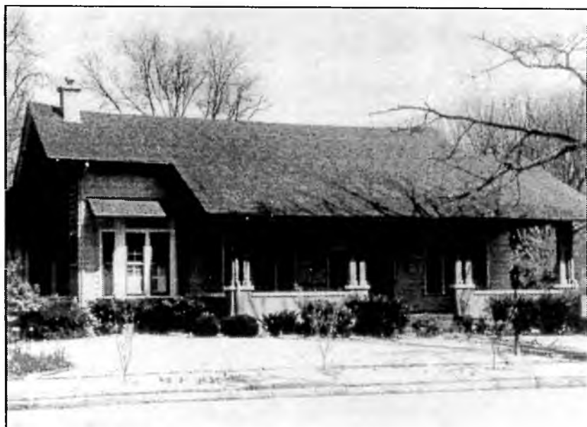
Fig. 5 In 1909, Huntsville architect Edgar Love designed this fine early bungalow at 531 Franklin Street. Notice the kick of the roof-ridge ends—a refinement found in at least one other Huntsville bungalow. The zigzag roof and bay window give this bungalow an informal and welcoming air. Courtesy Lynn Jones.
