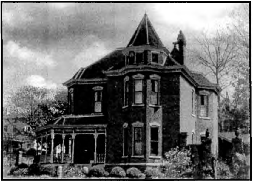
Fig.1 This 1899 house at 308 Eustis Avenue illustrates that the Victorian styles held sway right up to and partly into the 20th century. This Eastlake-style house is of unusually fine detailing and workmanship. The pressed-brick walls have extremely tight, barely invisible mortar joints, for the objective of brickwork of this period was for the wall to appear monolithic. The architect is unknown. A nearby church with similar brickwork has recently had its joints gouged out and wide, white mortar joints installed, as a sad revision to the original beauty of the walls. Courtesy Lynn Jones.
