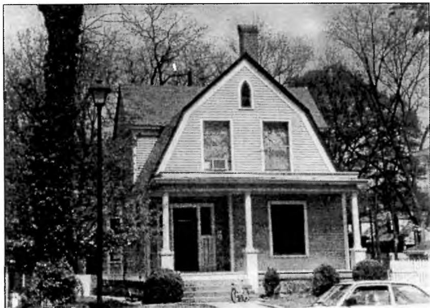
Fig.2 The architect Herbert Cowell designed this 1901 Dutch Colonial house at 603 Franklin Street, using a Dutch-Colonial gambrel roof combined with late-Victorian massing (vertical, narrow, irregular). A small Gothic vent is in the gable. The windows are quite wide and squarish in proportion, unlike those in the Victorian styles. A balustrade once ran along its porch roof, as evidenced by the base for it, and there may have been a balustrade also at the porch floor level that ran between the masonry piers that support the porch columns. Courtesy Lynn Jones.
