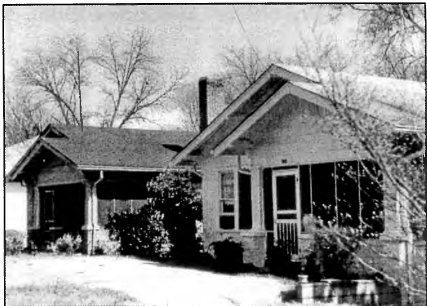
Fig.8 This pair of small identical bungalows at 430 and 432 Locust Avenue were built in 1923. They were probably built from stock plans on speculation, as many houses were in the 1920s boom period. The front porches were likely enclosed later, for screened front porches are not common in this period. The builder of these houses is unknown. Courtesy Lynn Jones.
