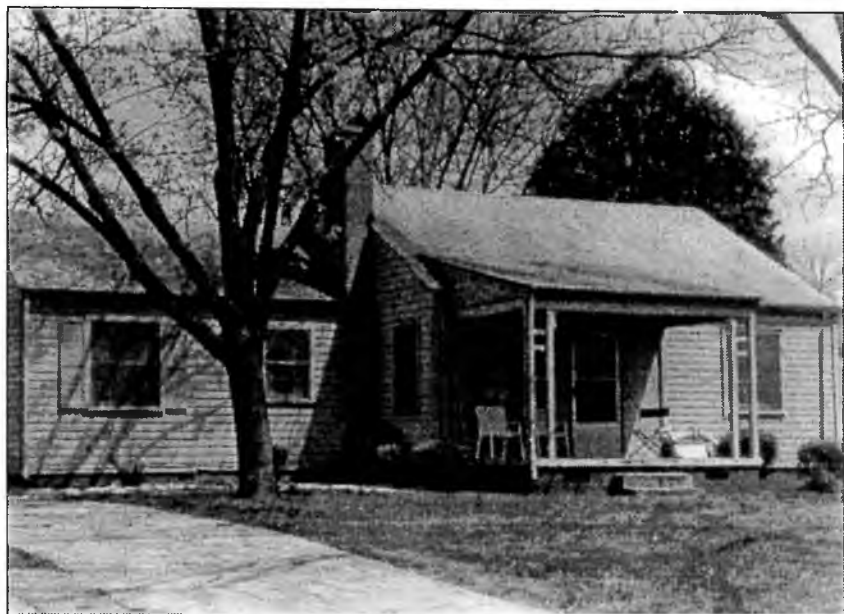
Fig. 13 A large subdivision of houses similar to this house on Sewanee Road was built in the early 1940s during World War II to house Redstone and Huntsville Arsenal workers. Its style is derived from old New England cottages, except with a front porch added, and thus could be called a Cape Cod Cottage revival style.
