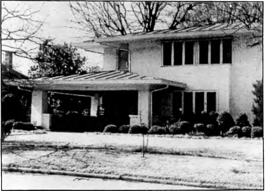
Fig. 7 Huntsville has two examples of the Prairie Style. One of them is the 1919 house at 709 East Randolph Avenue—a bungalow substyle developed in the Chicago area. Not only that, but it is closely patterned after a house designed by the famous architect Frank Lloyd Wright, published in the April 1907 Ladies' Home Journal as "A Fireproof House for $5,000" (Brooks 123). There seems little doubt that this house was derived from Wright's design, the only significant difference being the large entry porch rather than Wright's trellis and terrace shown beside the entry. The contractor was J. Nathan Williams. Courtesy Lynn Jones.
