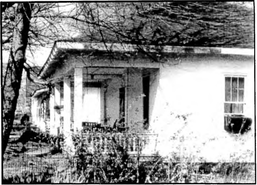
Fig. 10 These mill-worker's rental houses on north Meridian Street were probably built in the early 1920s by Lincoln Mills. While small and modest, the houses display the bungalow characteristics of wide, low eaves with exposed rafter-ends, wide front porch and rough-cast stuccoed walls. In its squarish hip-roofed form, these bungalows are actually closer to the original Bengali bangala than most of the more elaborate Swiss-influenced versions. Courtesy Lynn Jones.
