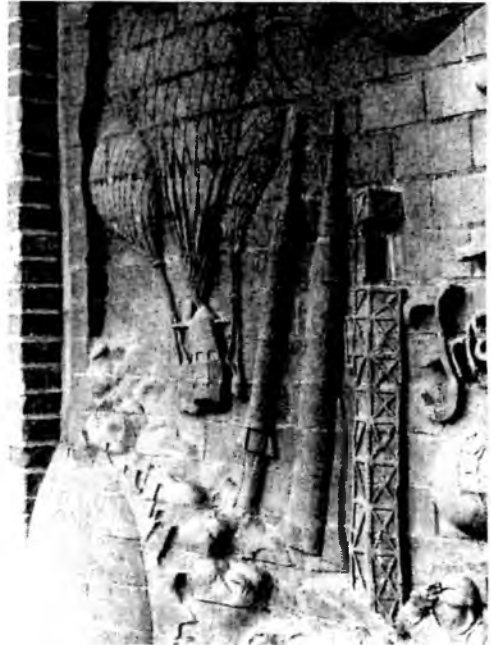
(25) General Shale Brick Co. Office, Whitesburg Drive, 1980's. A carved-brick mural produced by gouging the soft unbaked bricks into the desired profiles, firing them, and laying them up like a conventional brick wall (more tricky than it sounds).
