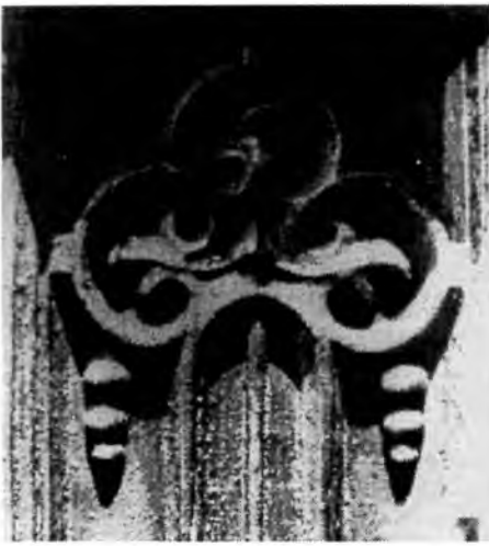
(4) The Church of the Nativity, 1859. Detail of ornament cast into the Gothic-Revival gatepost. This gatepost is an example of mid-19th century industrialization; an identical design can be found at a Mobile cemetery. Cast-iron building components in 1859 could be picked out of catalogues just as most parts for buildings are today.
