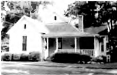
808 Ward Ave.—Simple Victorian wood-frame homes retain the varied massing and L-shapes of more elaborate Victorians. The exterior details are simpler and restricted to the use of shingles or siding. This updated version is aluminum sided. Photo Susan Bridges.
