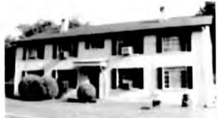
1122 Wellman — Apartments provided landlords with suburban income. The German Bauhaus influence can be seen on this 1930s building in the large casement windows, simple box shape, and smooth exterior. The shutters and slope to the entry overhang are probably later additions. Photo Susan Bridges.
