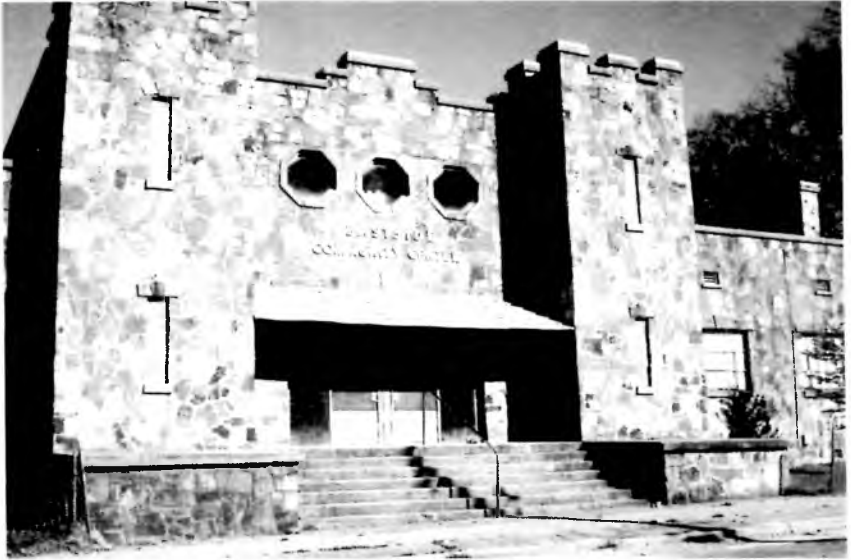
The Eastside Community Center, Old Town—Threatened by road development and expansion, this crenellated, castle-like building is a prime example of uncoursed random stone work used for public buildings in the early 1900s. Repointing and the stone's durability have helped the structure weather many uses.
