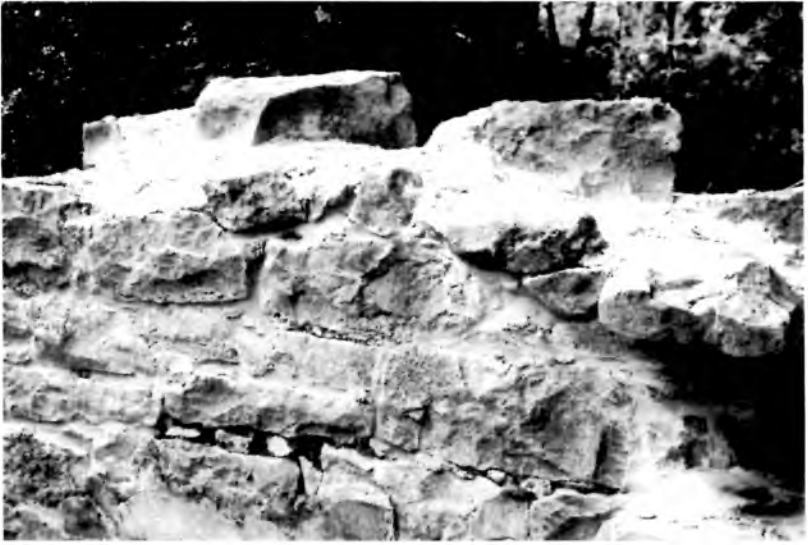
Monte Sano (Chapman) Dairy—The preserved ruins of the roughly-coursed, undressed limestone walls illustrate the vernacular use of stone. The thick stone walls also helped the dairy maintain cool temperatures for their products. Photo by Diane Ellis.
