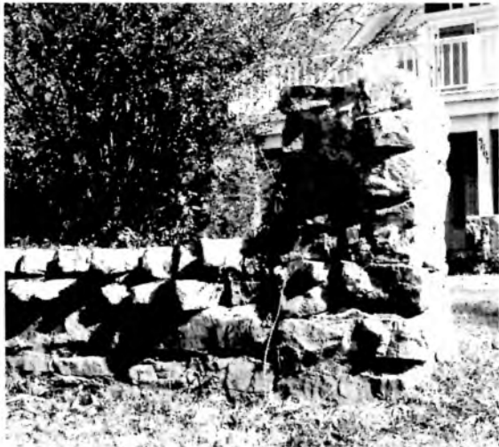
5607 Panorama—This rubblework fence in front of a stone/frame house incorporates found shapes as well as stone roughly cut for the top two courses of jagged, pointed projections.
