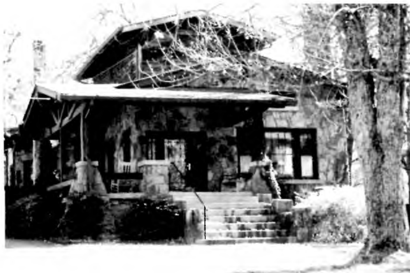
1711 Monte Sano Blvd.—The Orendorff home is an Arts and Crafts two-story stone and wood structure that incorporates random range ashlar on the main home and rubblework with slight coursing for the piers that support the porch and front steps. Photo by H. Cross.
