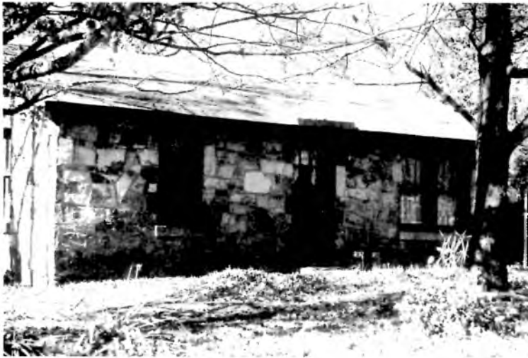
3618 Fearn—Random range rubblework on a solid stone wall home. The stone window sills are sloped away from the window and contain a drip edge (a shallow groove underneath the front edge) so that water drips to the ground instead of running back toward the stone where it can wear away mortar. Photo by H. Cross.
