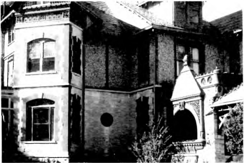
Kildare—The O'Shaughnessy home displays a rusticated foundation and porte cochere piers, dressed ashlar with painted brick quoins, carved stone details around peaks, and a slate roof. The third floor facade is composed of stucco and pebbles. Photo by H. Cross.
