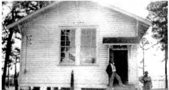
Mt. Carmel Elementary School—North or south end of building with entrance and cloak room windows. Two teachers pictured suggests this is a two-room building. Note electric wires. 1951. Courtesy H/MCPL.
