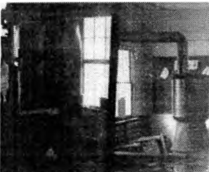
Toney Baptist Church School—Interior showing dangerous exposed stove flue and lack of lighting and desks. 1951. Courtesy H/MCPL.
