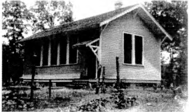
Mt. Lebanon School—One-room building with painted exterior and side entrance. Note Craftsman details such as brackets and exposed beams under wide overhangs. 1923. Courtesy Fisk University.
