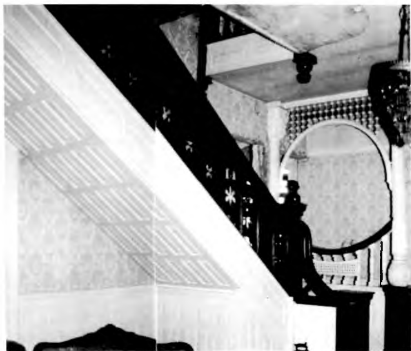
Figure 6: Entry hall before renovation. Note black and white paint on staircase.
