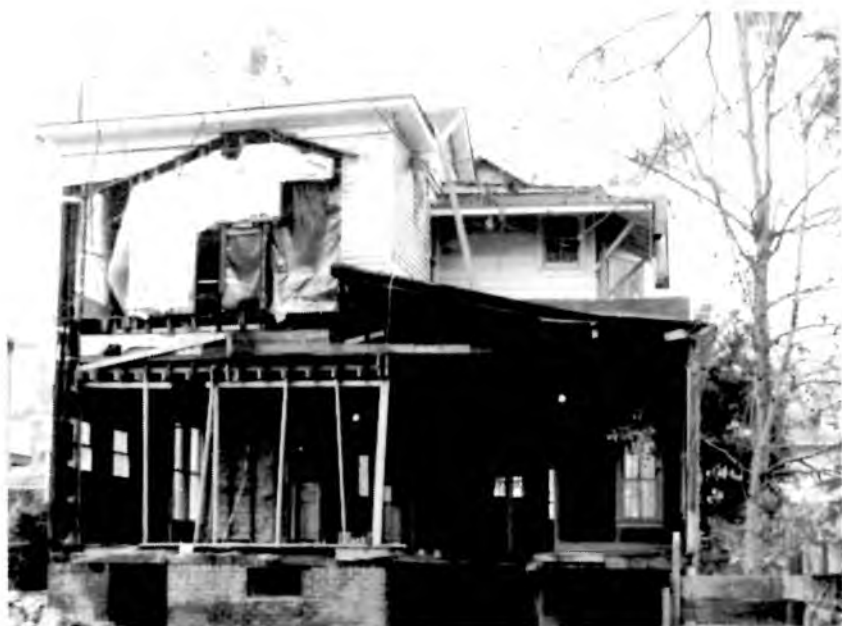
Figure 4: West rear during 1997 restoration, after removal of “makeshift addition.”
